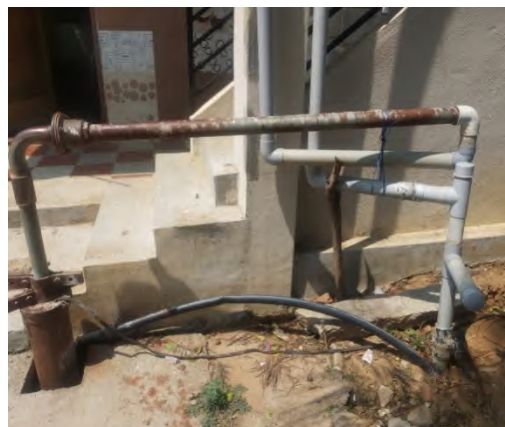
Rainwater used to recharge the borewell
